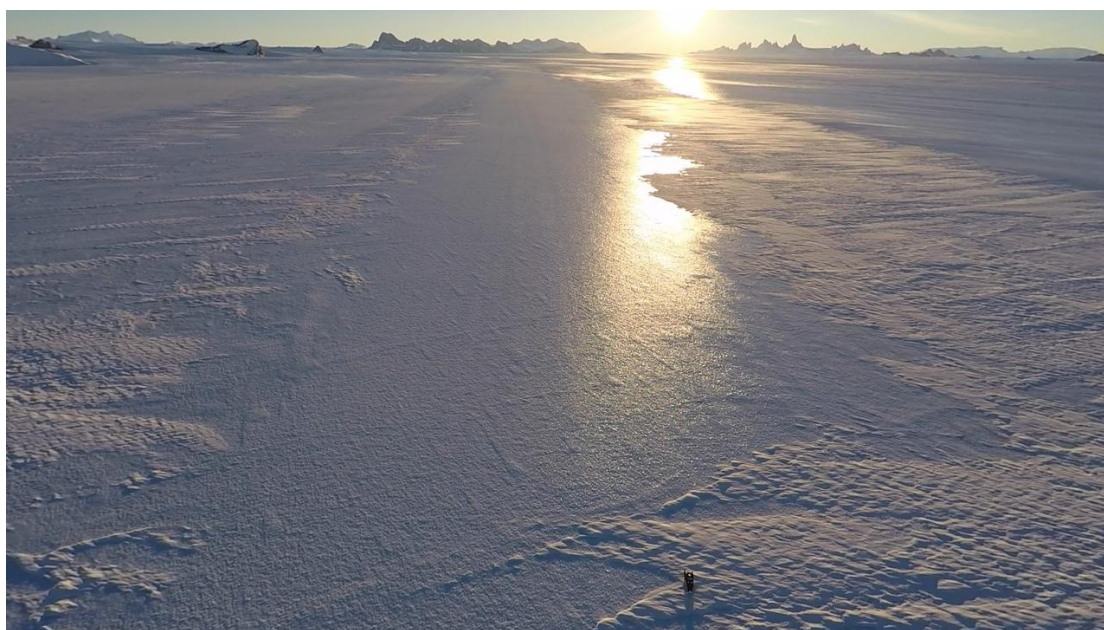
Image 5. The proposed Wolfs Fang Runway looking South. The slight bumps on the surface are white ice deposits formed by melt/refreeze processes under snow drift deposits which have since ablated away. The orientation suggests formation under South Easterly winds.
